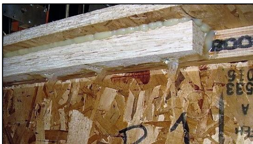
Figure 4: Example of sufficient “squeeze-out” behavior (left); West System® Six10® Thickened Epoxy Adhesive (right).
