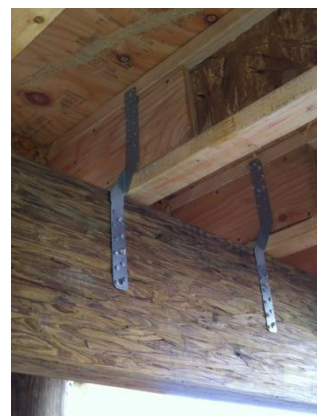
Figure 8: Joist to Beam Connection Detail.
