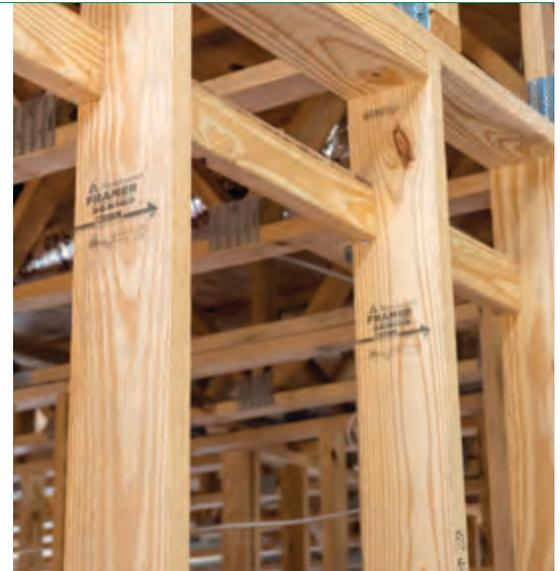
Weyerhaeuser Framers Series lumber is mechanically graded to virtually eliminate warping, and each board comes with the crown clearly marked to speed up installation. With lumber like this, framing goes up fast, crews won't spend valuable time culling, and there's less material waste when the job is done.
