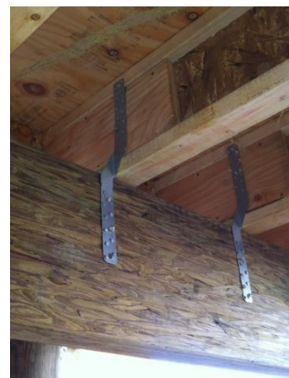
Figure 8: Joist to Beam Connection Detail.
